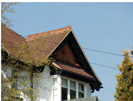
Picture 2.61 Tile hanging on gable ends, Green Lane
