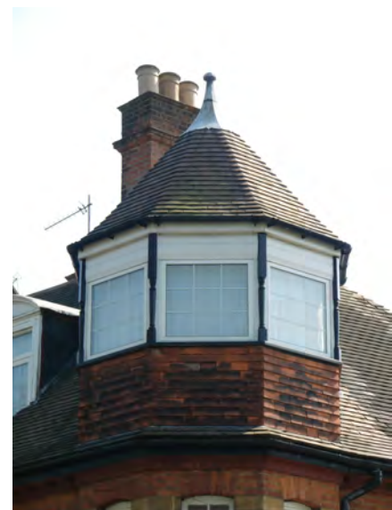
Picture 2.48 Corner turret at locally listed no. 107 Stanmore Hill
