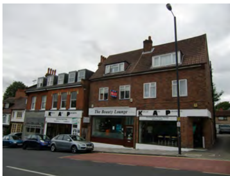
Picture 2.42 Shopfronts that present opportunity for good quality replacements ie 83, 85, 87 and 87b Stanmore Hill
