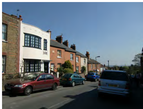
Picture 2.54 Small scale cottages, Green Lane
