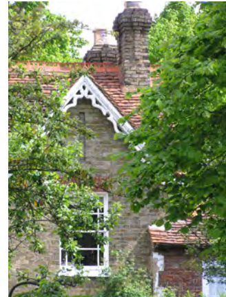
Picture 2.65 Decorative timber bargeboards, and clay ridge tiles and historic timber sash on a property along Stanmore Hill
