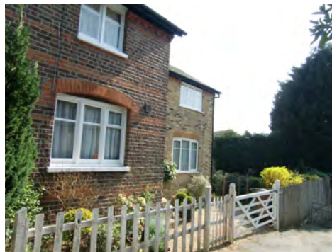
Picture 2.67 Timber casement windows and brick banding detail on Park Cottages on a small side road off Green Lane
