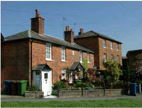
Picture 2.8 Grade II listed 1-5 Pinnacles Place and Park House
