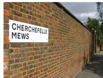
Picture 2.25 Important historic brick wall of Cherchefelle Mews fronting public highway, lower reaches of Green Lane
